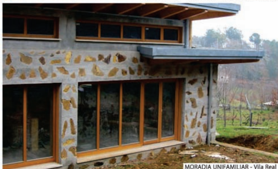
MORADIA UNIFAMILIAR - Vila Real
